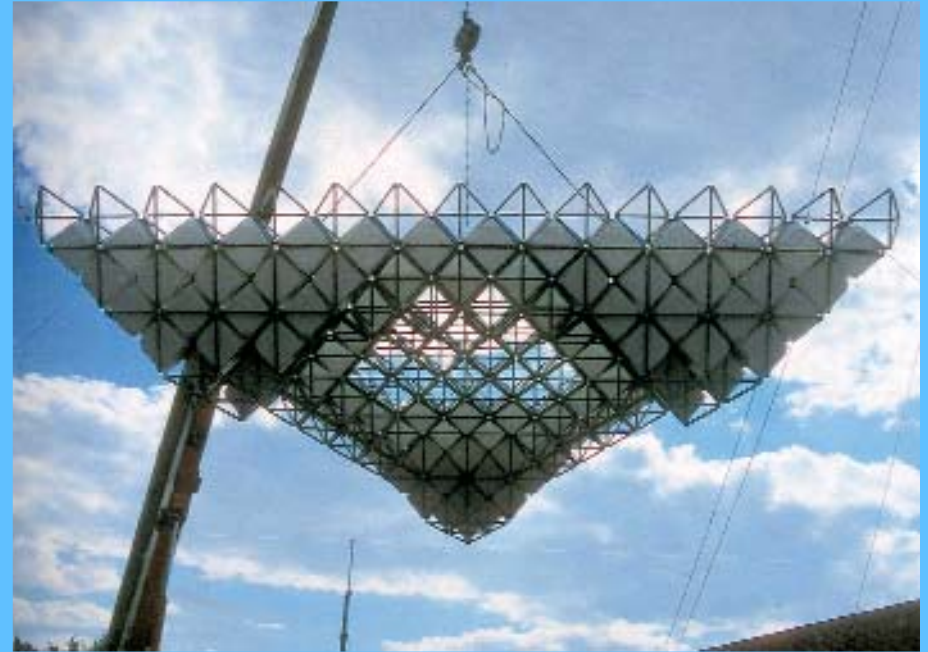
The FLOATING PLATFORM is launched with a crane.
